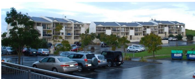
Figure 6. Internal view of the Albany case study development. The photograph shows the extent of surface car parking and poorly positioned waste disposal facilities (source: authors).
