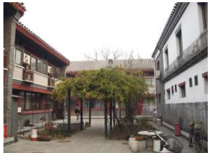
Figure 5. A new courtyard at Beijing Nanchizi Chinese-style new courtyard housing estate. Photo: Donia Zhang 2007.
