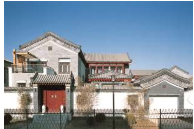
Figure 13. A closer view of a Guantang courtyard garden villa with traditional enclosing walls, gate, and modern garage. Source: Beijing Institute of Architectural Design 2014.
