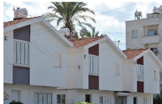
Figure 19. The Clean, abstract and White surfaces for Efruz Housing (Image by Author, 2016).
