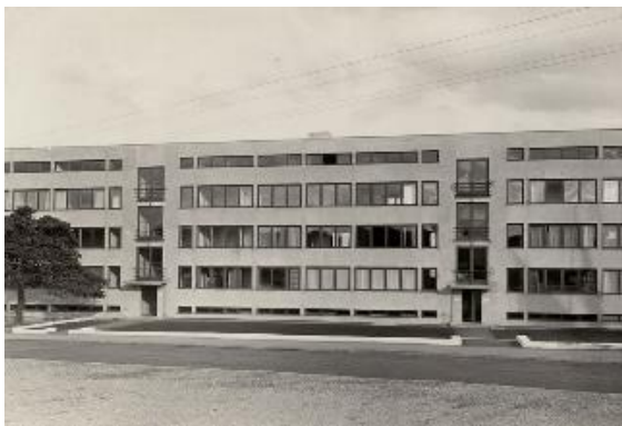
Figure 5 . Ludwig Mies van der Rohe Weissenhof Housing Project. (Pevsner, 1968).
