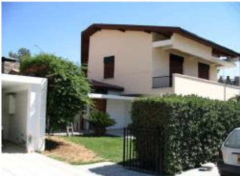
Figure 26. Ferdi Macit House MACIT FERDI HOUSE, NICOSIA 1961 ( D.Celik,without date).
