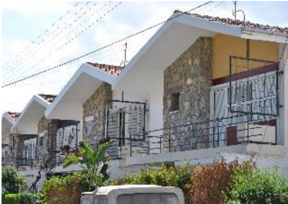
Figure 20. North Elevation of Efrus House (Image by Author, 2016)
