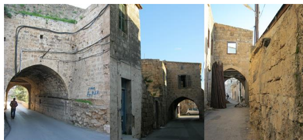
Figure 6. Street in the traditional quarter of Gazimagusa (Photo by author. 9th Januar 2016, Walled Ctiy).
