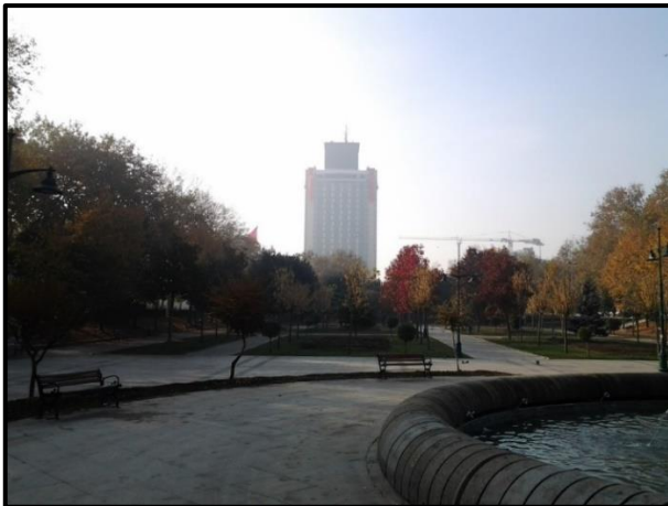
Figure 5. A view from inside the park, with the Marmara Hotel on the background (authors' archive, October 2013).
