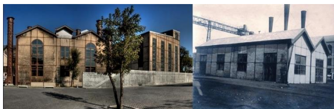
Figure 15. Adaptive reuse in Santralistanbul previous and new building.
