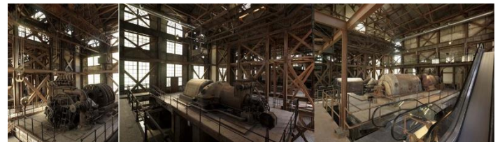
Figure 14. Less intervention and the visibility of structure from inside.
