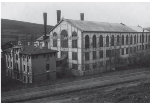
Figure 9. Silahtarača Power Plant, view of the first machine room and administrative headquarters (Adopted from (Brangar, 2004))
