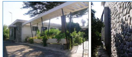
Figure 21. Using Iron forks in the right and exposed stone facade in the left (Hera, 2010)
