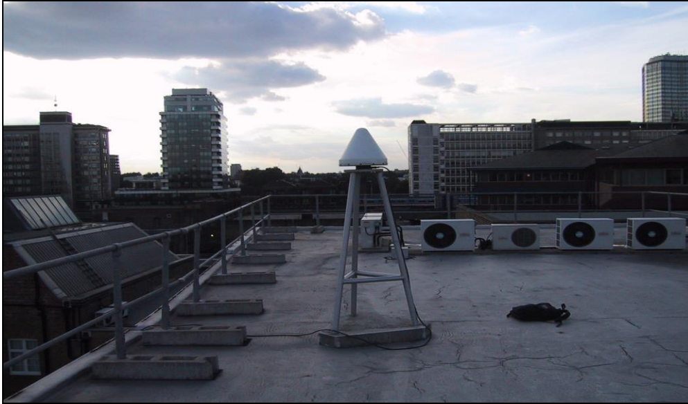
Figure 11: Multipath Environment (Ordnance Survey Headquarters, Central London). Note the air conditioning vents located on the centre-right of the figure.
