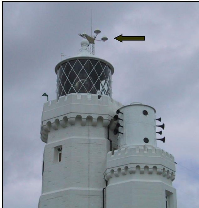
Figure 22: GPS Antenna, SCP1
