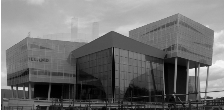
Figure 11: Today's state of construction.
