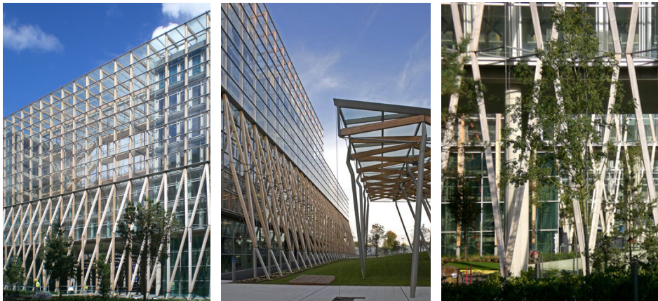
Figure 5,6 and 7: Double façade of the Elm Park Development..
