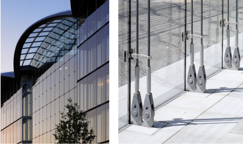
Figure 6: Lufthansa Aviation Center, Frankfurt
