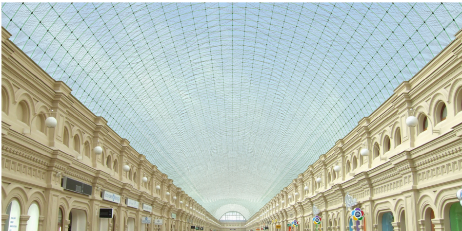
Figure 19: Artist's impression of the developed system, based on the GUM-facades (14 m span)
