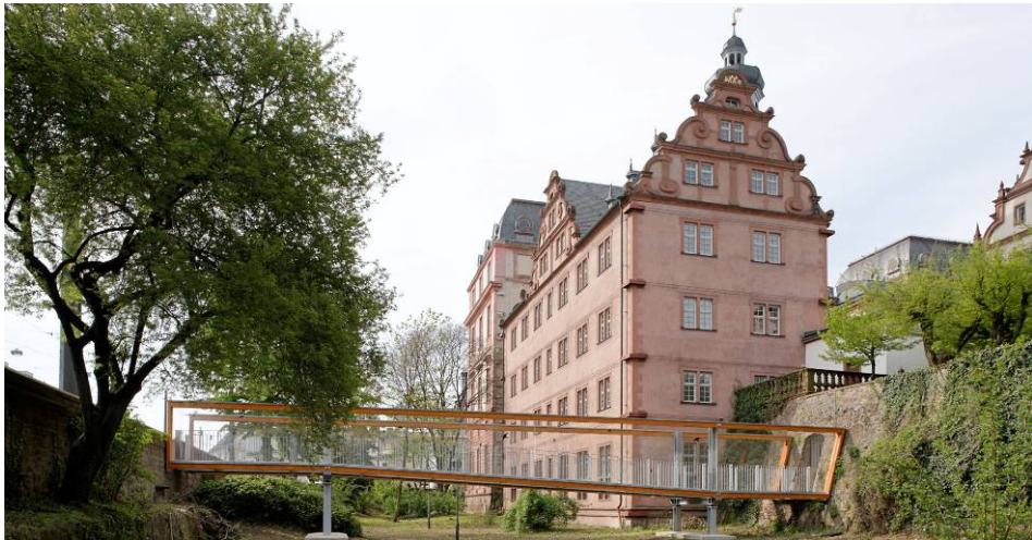
Figure 11: Prototype – palace moat bridge in Darmstadt, Germany.
