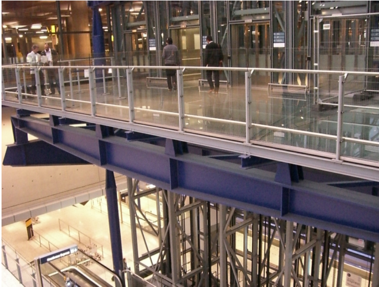
Figure 1: Heathrow Express Lift Landing, Terminal 5, Heathrow Airport
