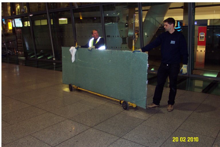
Figure 5: Removing shattered top sheet
