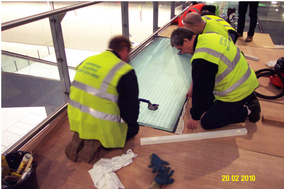
Figure 7: Installing new top sheet
