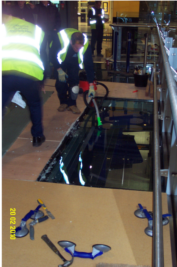
Figure 6: Cleaning remaining structural laminate
