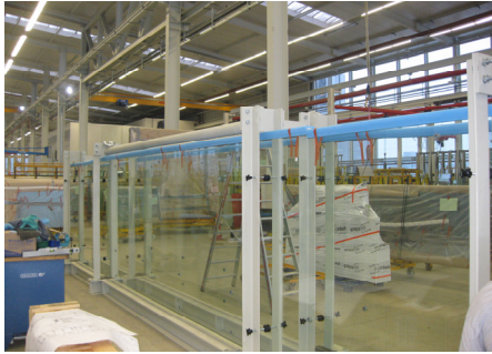
Figure 9: Glass balustrade supported in temporary steel frame.
