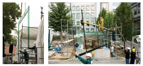
Figure 8: Glass frame erection.
