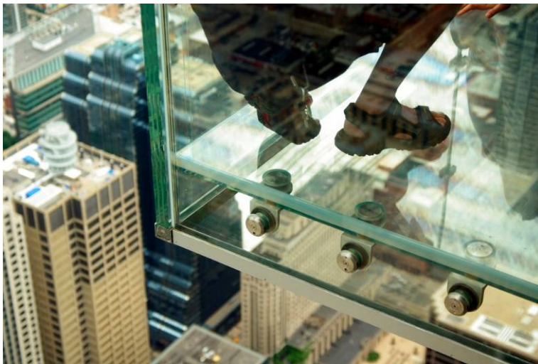
Figure 9: Typical glass connections. Heat tape strips are located inside the aluminum edge at the bottom. [3]
