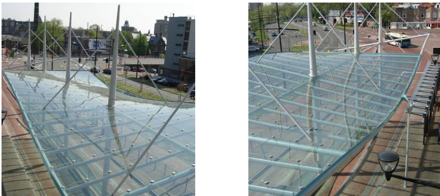
Figure 14: Glass roof from above
