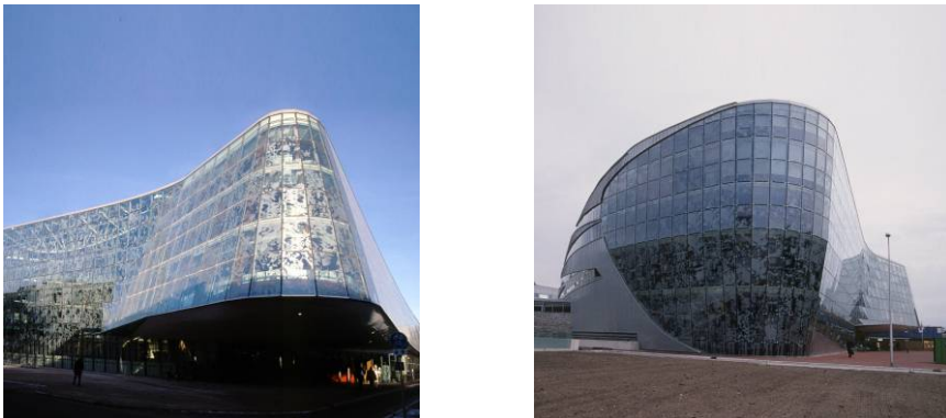
Figure 6 : Overall view and detail view of the town hall façade
