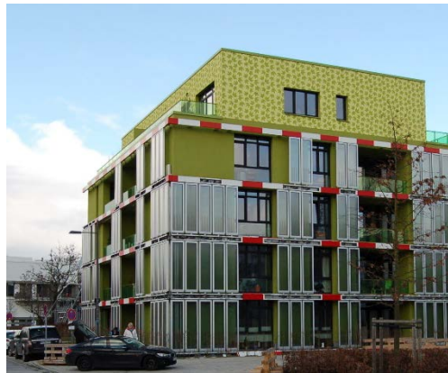
Figure 2: A bioactive facade installed at the BIQ- Algenhaus in Hamburg, Germany.
