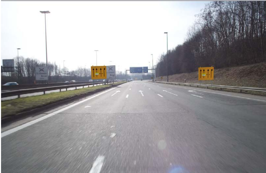
Figure 8. Interference between temporary and permanent traffic signs.
