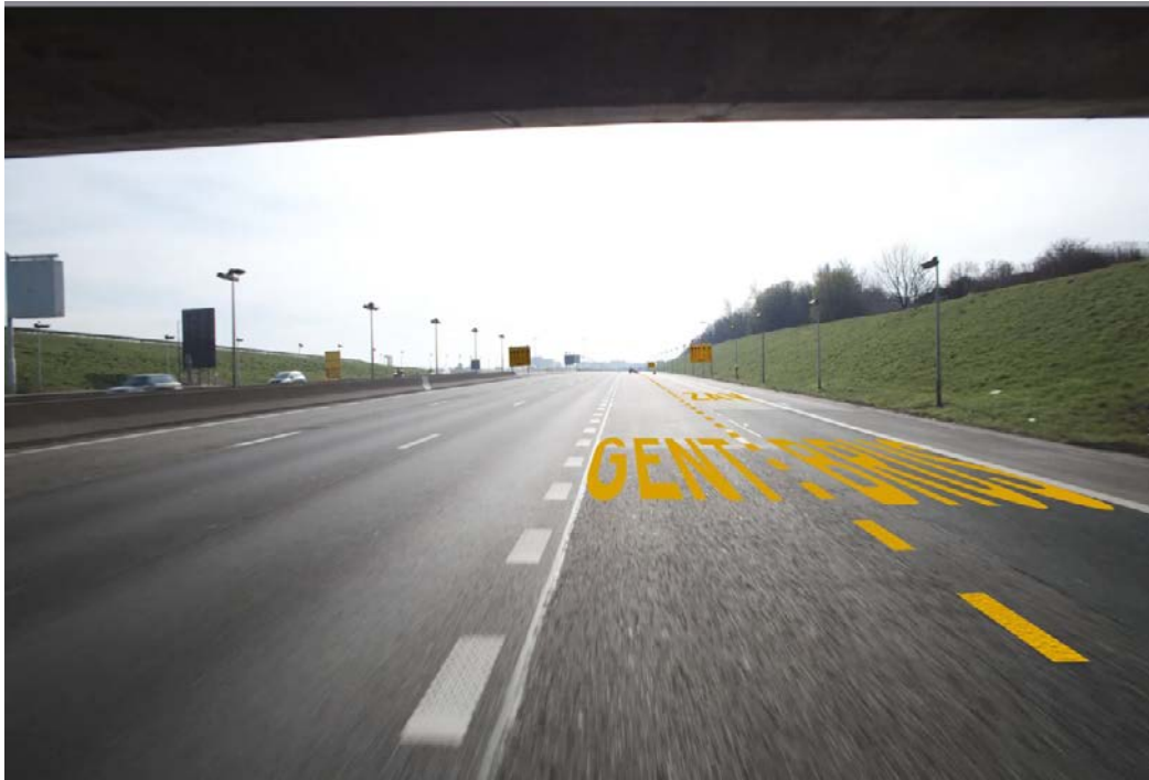
Figure 9. Temporary pavement markings with destination names.
