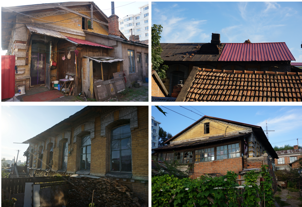
Figure 7 Environment of historic buildings
