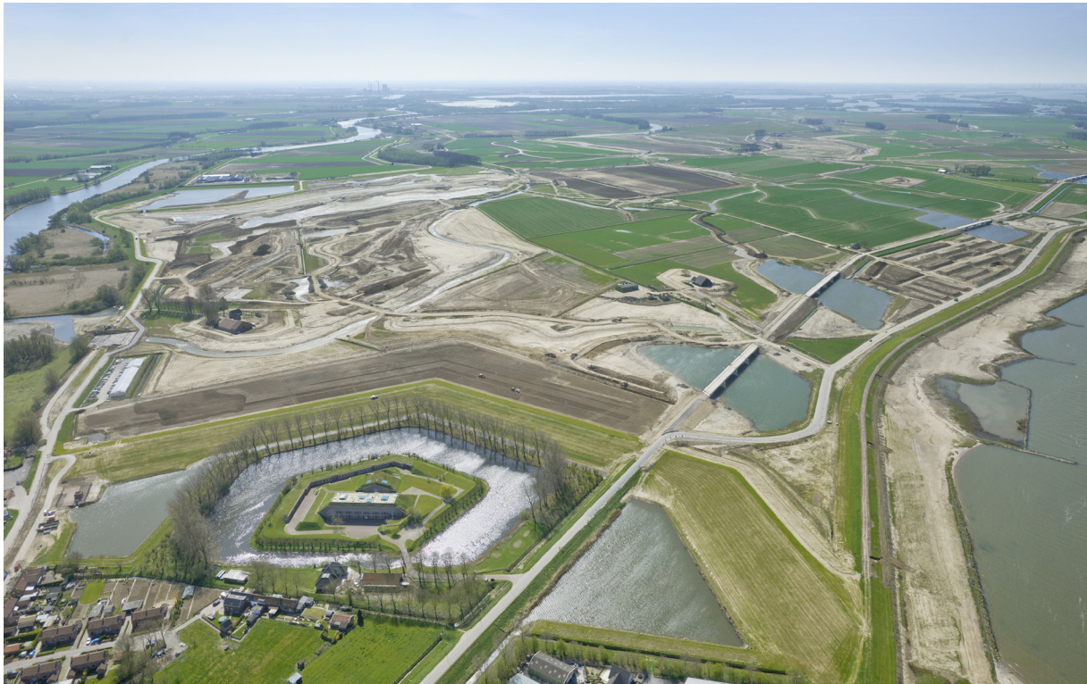
FIGURE 3 Aerial view of polder Noordwaard during reconstruction, 2015. Aerophoto Schiphol
