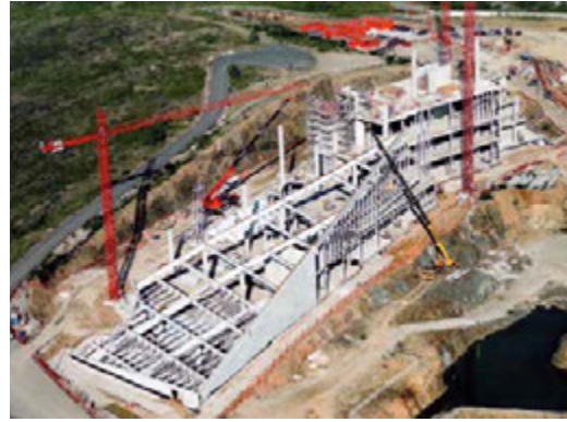
FIG. 6.4.2 central services under construction
