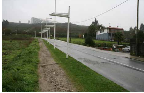
FIG. 6.3.2 ... a worksite abandoned after parliament ...
