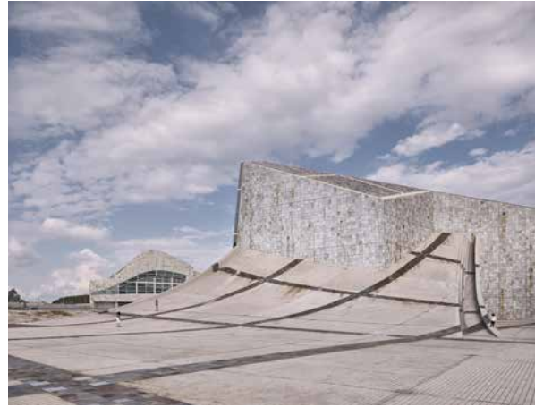
FIG. 6.5.1.16 Roof raising from central square to library
