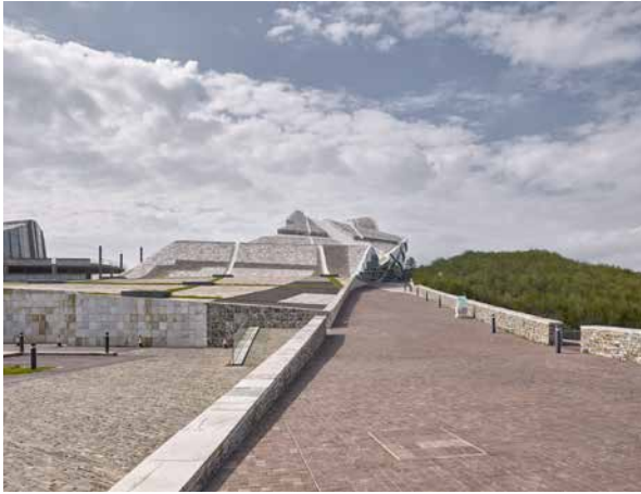
FIG. 6.5.1.15 North Eastern edge of Roof (Photos: Ariel Huber)
