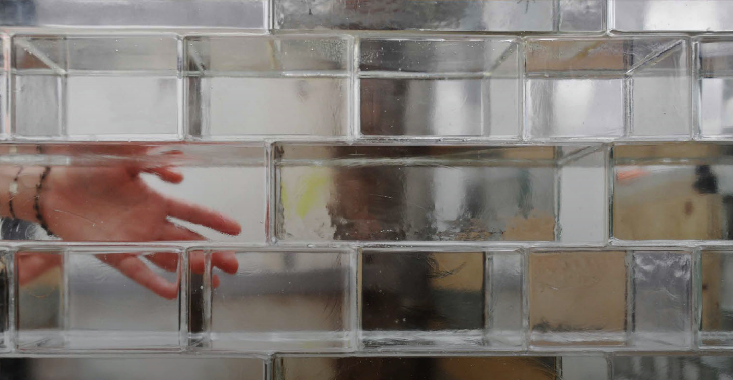
The two developed systems utilizing solid cast glass components. In this page: Adhesively bonded solid glass blocks. Next page: Dry assembled, interlocking cast glass components.
