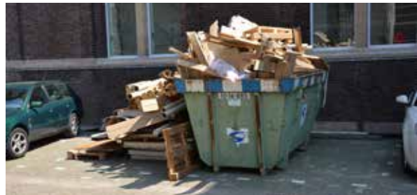
FIGURE 7.39 Dismantled and ready to be recycled TECH 02
