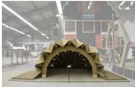
FIGURE 6.54 Open structure with the entrance arch fitted to the floor panel
