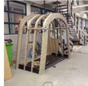
FIGURE 6.148 Partly realised prototype
