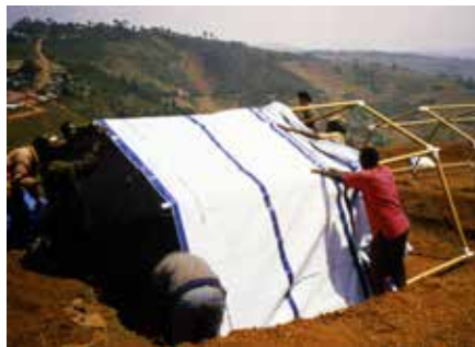
FIGURE 5.22 UNHCR tent with paper tube structure, Rwanda, 1999
