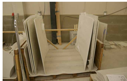
FIGURE 6.31 Finished cast panels for ring 1 and ring 2.
