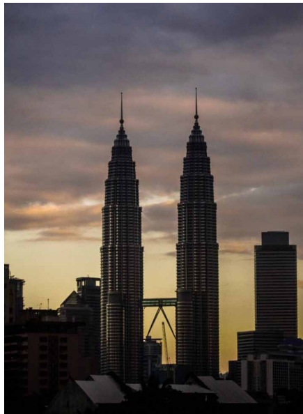
FIGURE 3.5 The Petronas Twin Towers. (Source: www.thisiskl.com )
