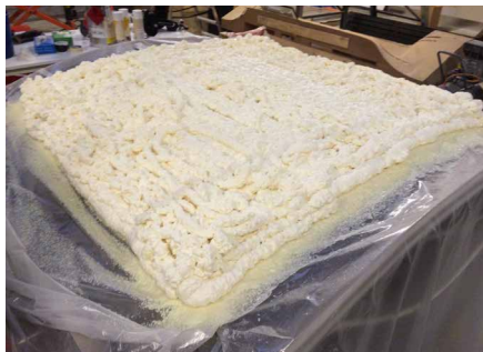
FIGURE 6.12 Curing the LDPU on the flexible table
