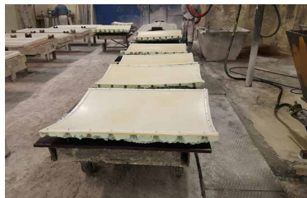
FIGURE 6.30 Intermediate moulds for ring 3-9 of the thin-walled GFRC hyperbolic shell before the first casting.
