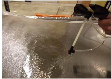
FIGURE 6.15 Applying the hard coat
