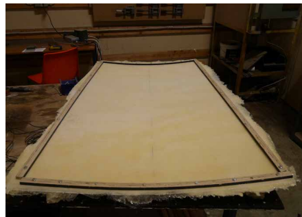
FIGURE 6.13 Fitting timber edges barriers on the mould
