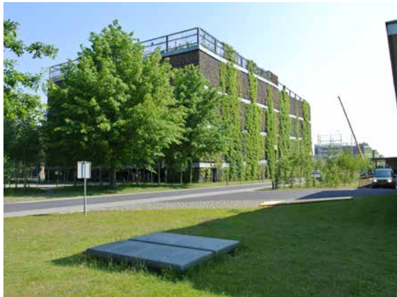
1 Parking garage in campus north
