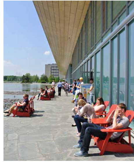
Figure 5.11 Central building housing amenities (2013)
