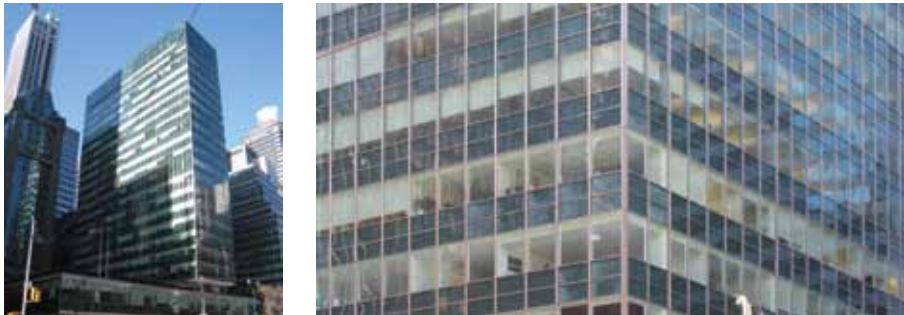
Figure 4 Street view and detail of the renovated Lever House, Skidmore Owings and Merrill, New York, 1952
