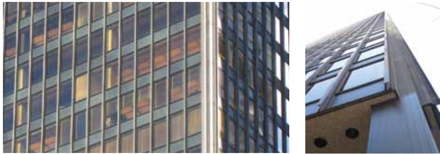
Figure 5 Detailed view and corner solution, Seagram Building, Mies van der Rohe, New York, 1958
