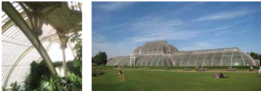
Figure 1 Palm House, Kew Gardens London, 1841-1849. Cast-iron columns and joists form the primary structure. The envelope consists of formed rolled steel profiles with bracing glass panes..
