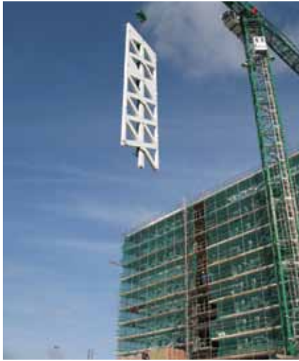
Figure 115 Assembly of the large pre-manufactured façade components
