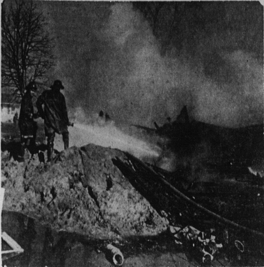
SMOLDERING RUINS — Holland firemen pour more water on the smoldering ruins of the Orlan Uitermark home, 454 West 21st St., where a gas explosion collapsed the wood frame structure Thursday seriously burning Uitermark and Ray Barrett, 41. Fire officials continued their investigation
