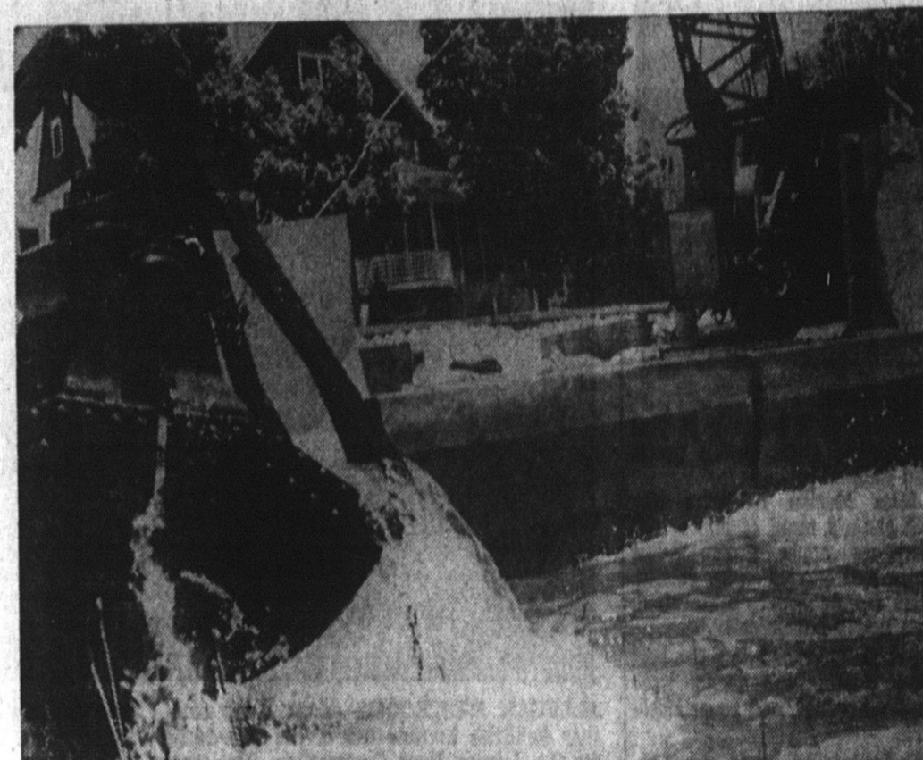
DEN UYL'S COTTAGE — Simon Den Uyl leads the effort to erect a sea wall. A total of 200 feet of the sea wall has already been constructed. The proposed wall is intended to be 700 feet long. Den Uyl's cottage is pictured in the background. (Sentinel photo)
