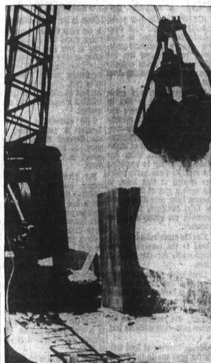
BACKFILLING WITH SAND — One of the operations involved in the construction and reinforcement of the experimental sea wall is backfilling. The crane is shown dredging sand from the lake. Also pictured is one of the wooden forms used in construction of the wall. (Sentinel photo)
