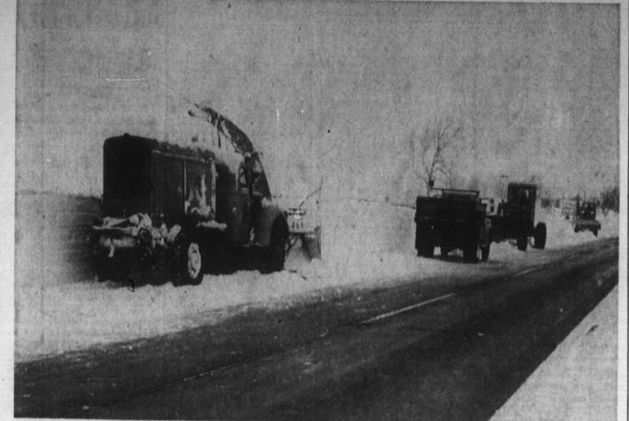
STILL CUTTING DOWN BANKS - A snow blower and other equipment of the Michigan State Highway Department continues work in cutting back the huge snowbanks on US-31 south of Holland. This heavy equipment slices down the bank and blows the powdered snow far into the fields. This service
