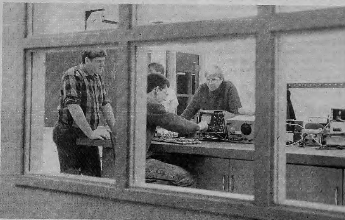
Several of the interior walls have had windows added, creating a sense of openness and breaking the monotony of solid-block construction.
