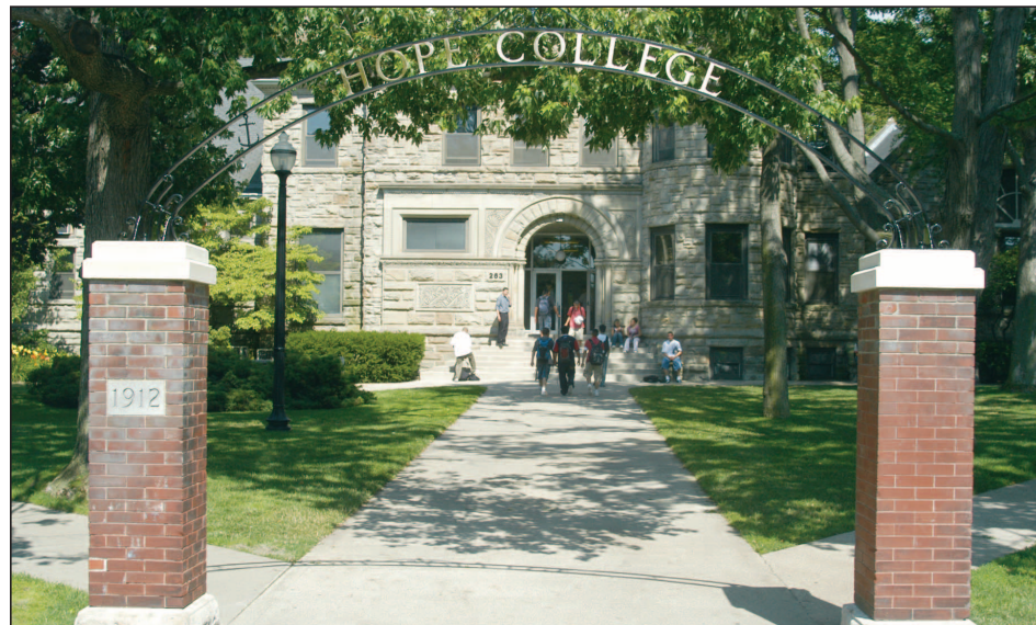
Certainly no one would wish for a truck to back into the landmark "Hope College" arch in front of Graves Hall, but the experience has ended in a good way. It turns out that the letters were brass, discovered during the course of repairing the historic nameplate. They now shine brightly for the first time in decades.
