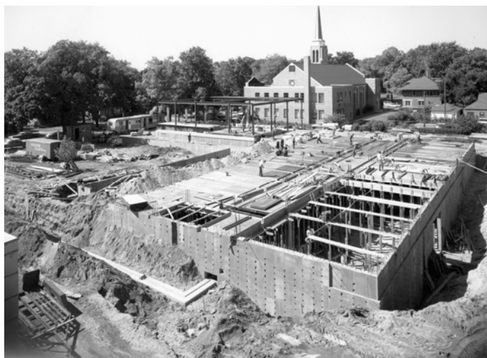
Construction began on the physics-math building in early 1962
