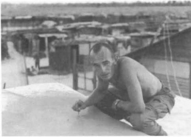
Fetters repairing damage
