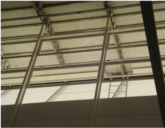
Figures 10 and 11. Walkways in great roof in sheds and equipment to facilitate the cleaning service located in the roof of the Sarah Hospital of Rio de Janeiro. Source: Marieli Azoia Lukiantchuki.
