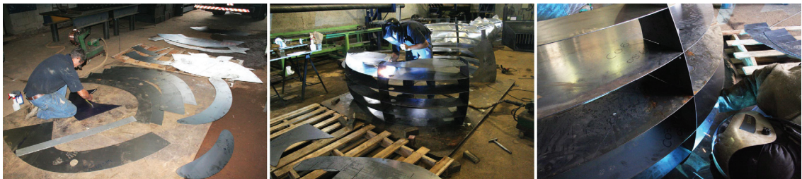
Figure 25. Assembling and welding process.
