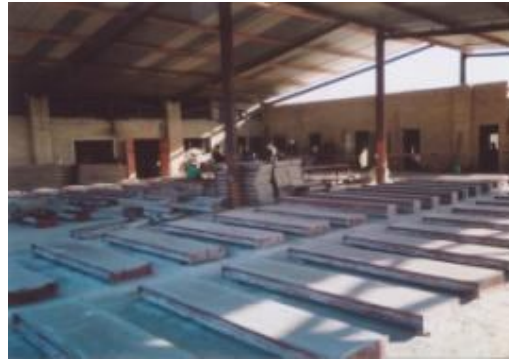
Image 8: On-Site Concrete Panel Factory
