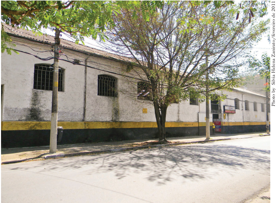
Photo 3 – Industrial Shed at 512, 550 Faustolo Street.
