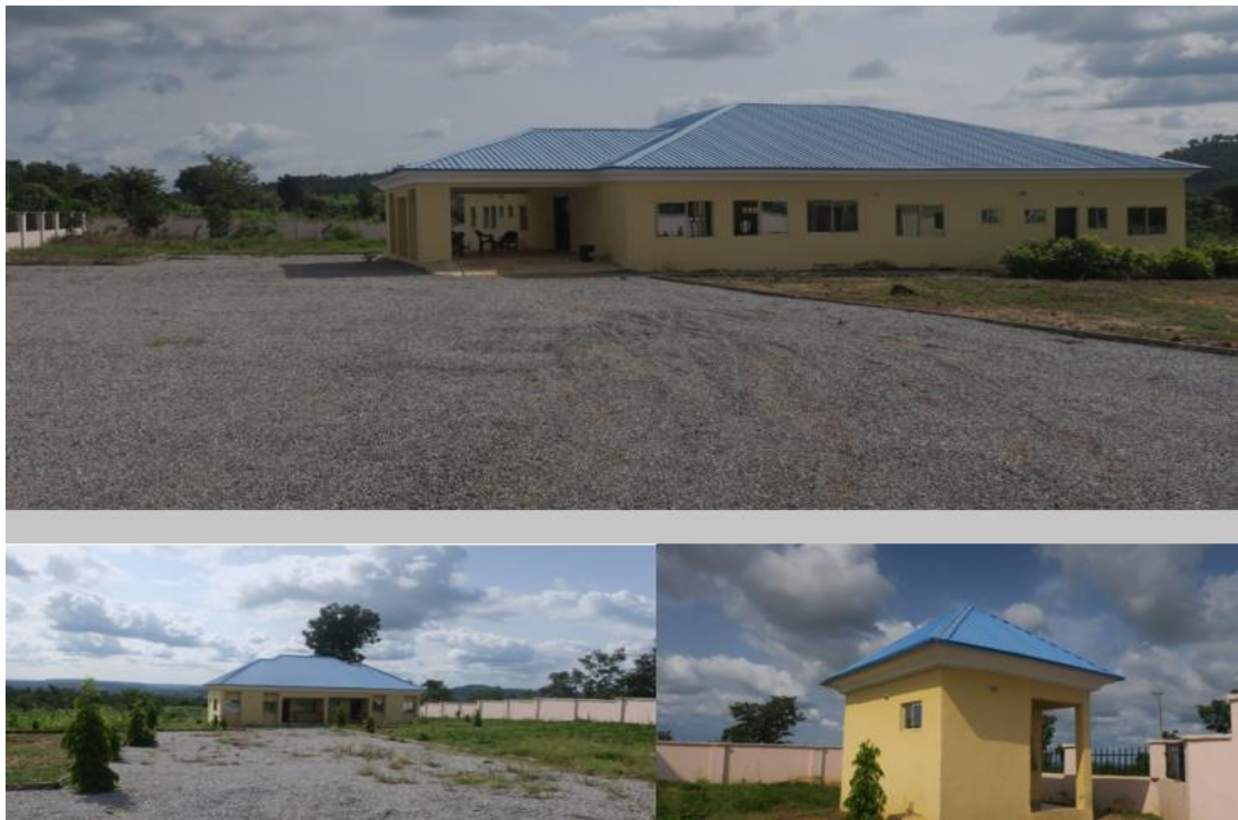
Figure 9. Pandagi Comprehensive Health Centre, Abaji Local Government Area Council, FCT (Photo by Author)
