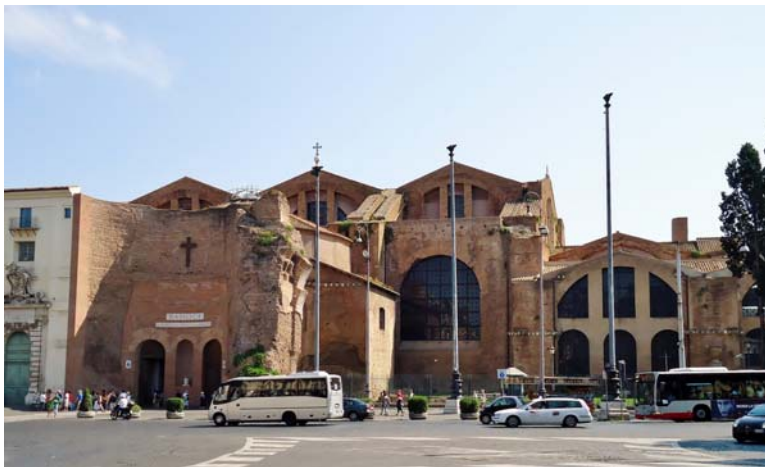
Figure 5: Facade of the Basilica de Santa Maria degli Angeli , facing the Republic Square. Source: author.
