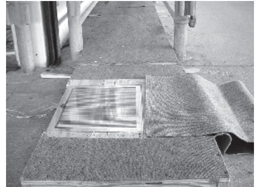
Figure 1 - Wooden platform inside restrain corridor
