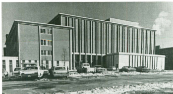
Unit 4 view from west
