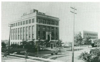
South Laboratory Building, 1927
