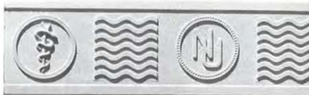
Detail of frieze, Hospital, Unit III, north, 1961.
