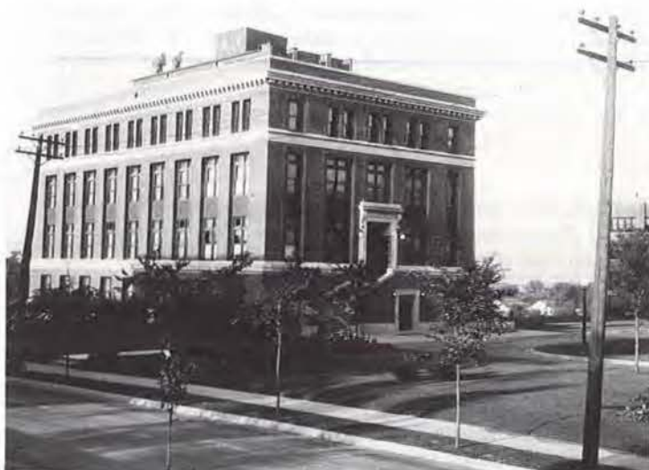
(Left) South Laboratory Building.
