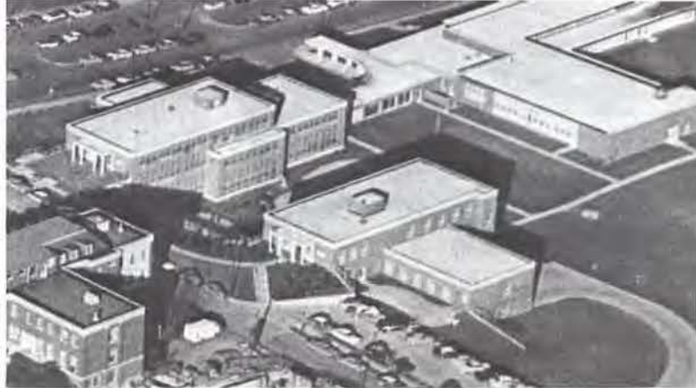
Aerial view, Children's Complex, from southwest, 1961.
