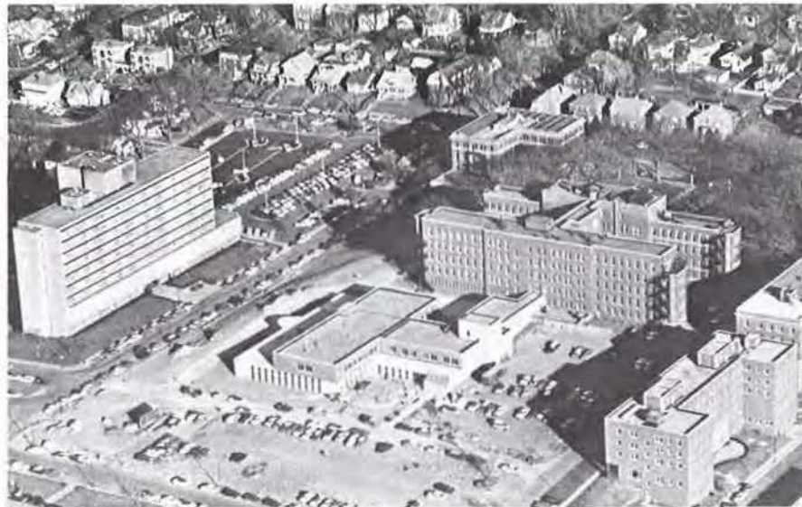
Aerial view, new hospi- tal, from southwest, 1961.
