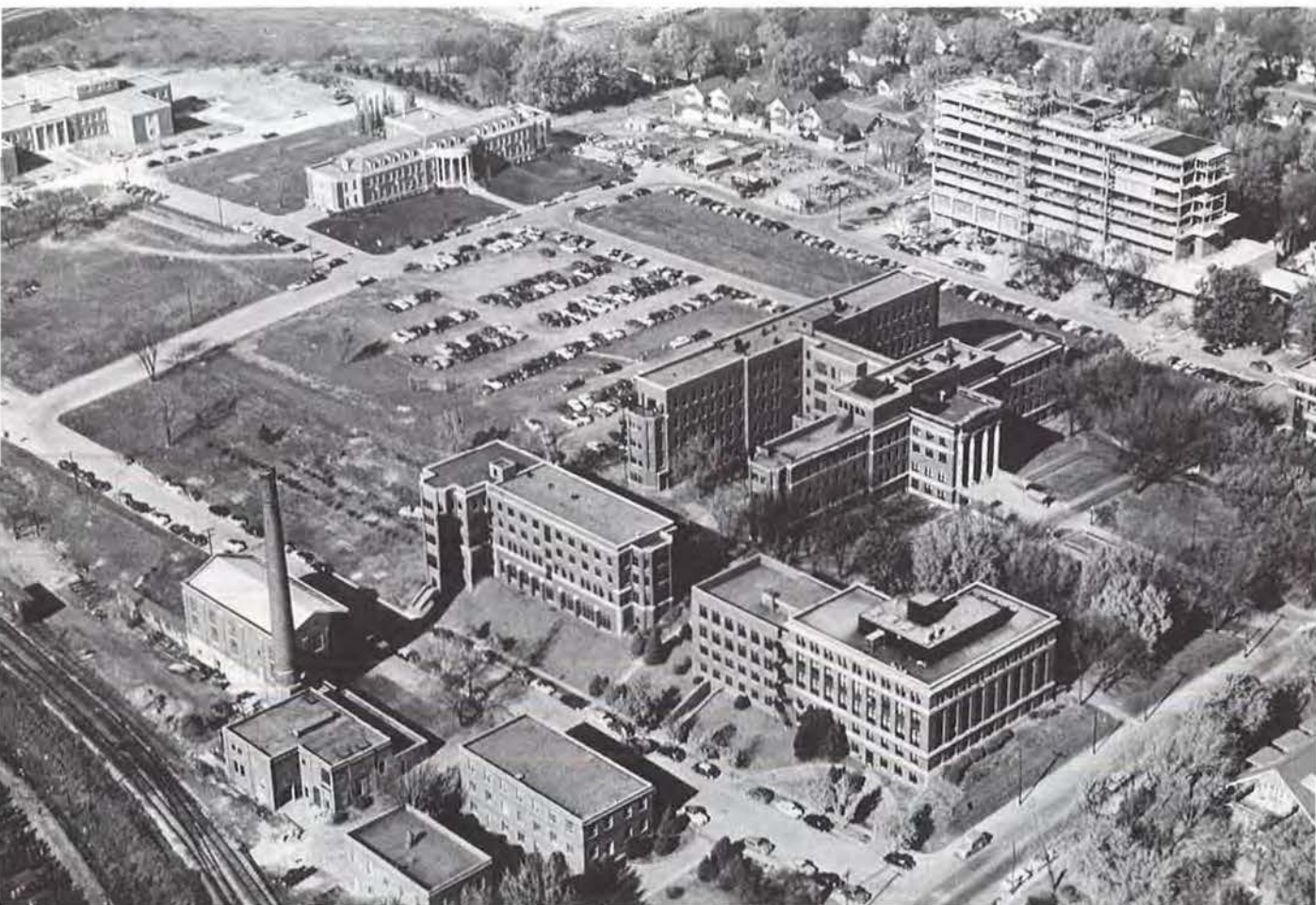
Aerial view, campus, Clarkson Hospital under construction, 1955.
