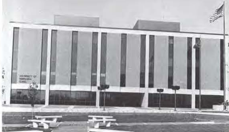
Clinic Building, dedicated October 2, 1977.
