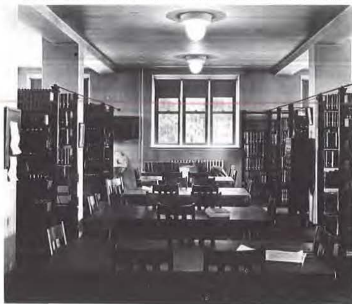
College library, second floor, administration wing, University Hospital.
