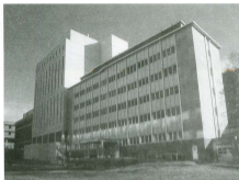
Figure 2. The Eppley Hall of Science with five floor addition
