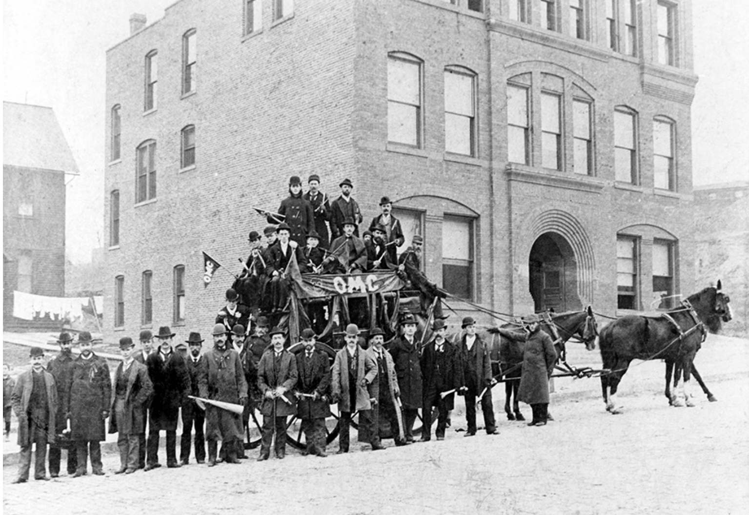
Medical Students from the classes of 1891-93 pose in front of the new medical college building. With a decade of success behind it, the college replaced the old frame structure with a new brick and masonry building on the same site.
